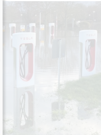
Tesla chargers at Woking @megbaynes
