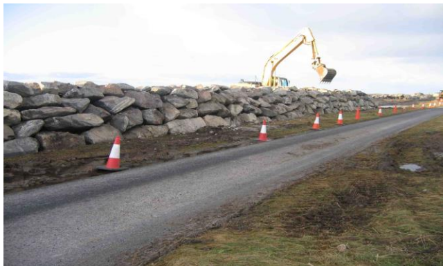
S. Uist, W. Isles, boulder protection of an easily rerouted minor road post 2005 storm, bypassed by storm wave overwash at sides as erosion continues.
