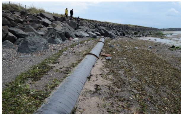
Prestwick, unprotected main wastewater pipeline emerges from boulder protection, itself inserted to prevent contaminated rubble from beach access.
