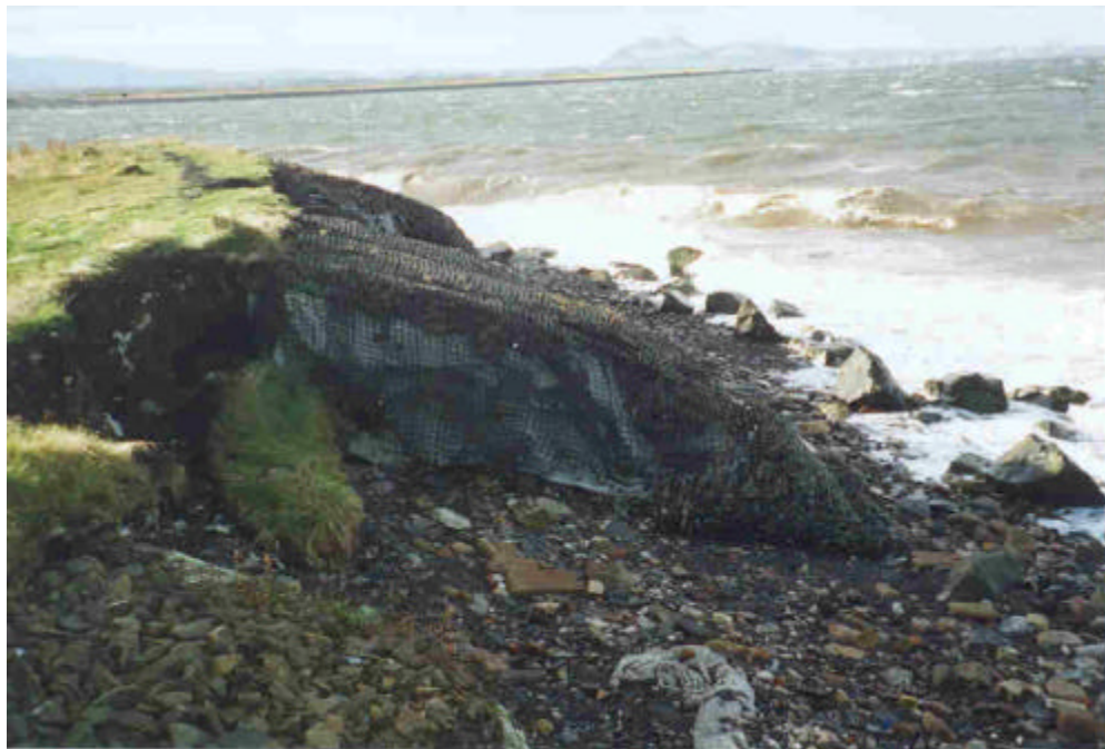
Observed Erosion and Damaged Gabion Defences at The Cast, Prestonpans.
