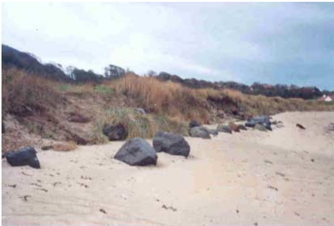
Plate 9.26 Defence No 38 North Berwick East Links (Dune Erosion)
