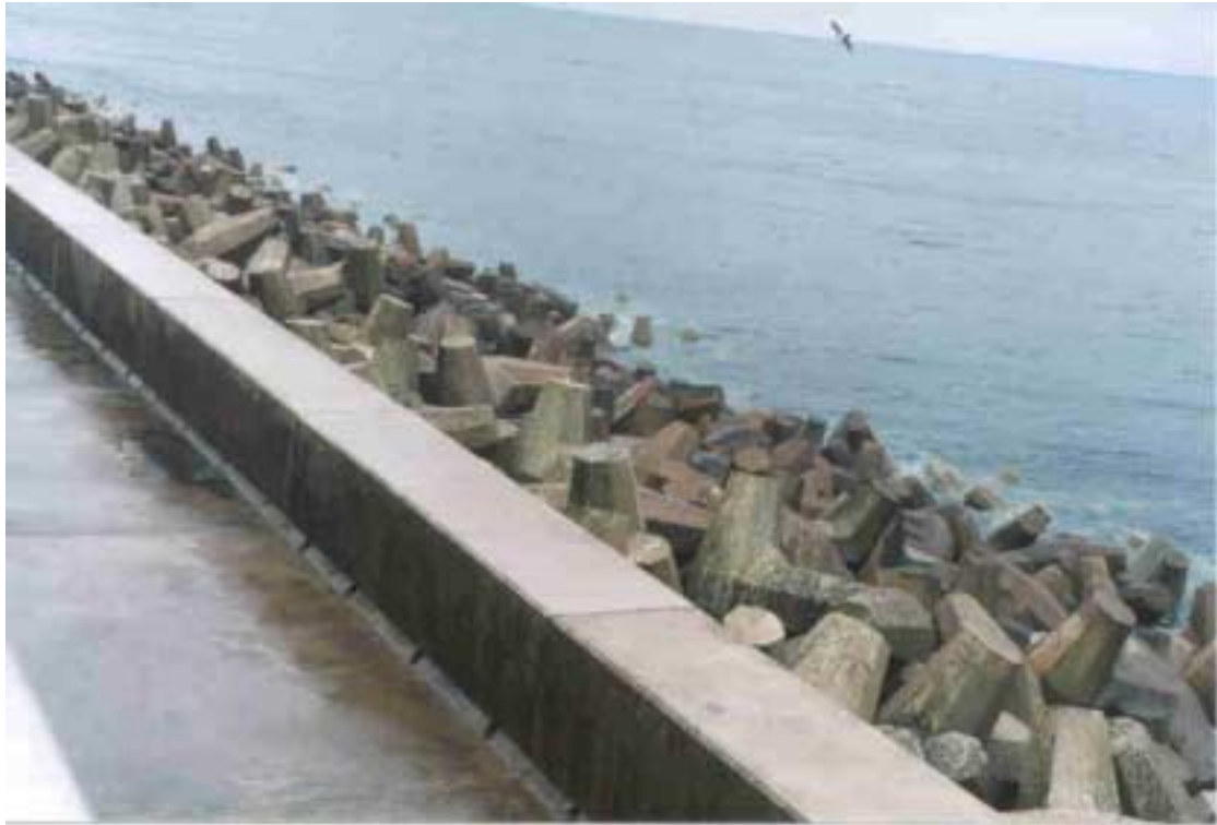
Plate 9.43 Defence No 58 Torness Power Station (Concrete Embankment protected by tetrapods)
