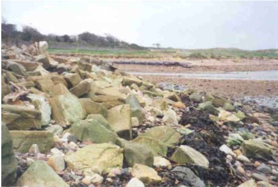
Plate 9.41 Defence No 56 Dunbar Golf Club East Links Rock Armour
