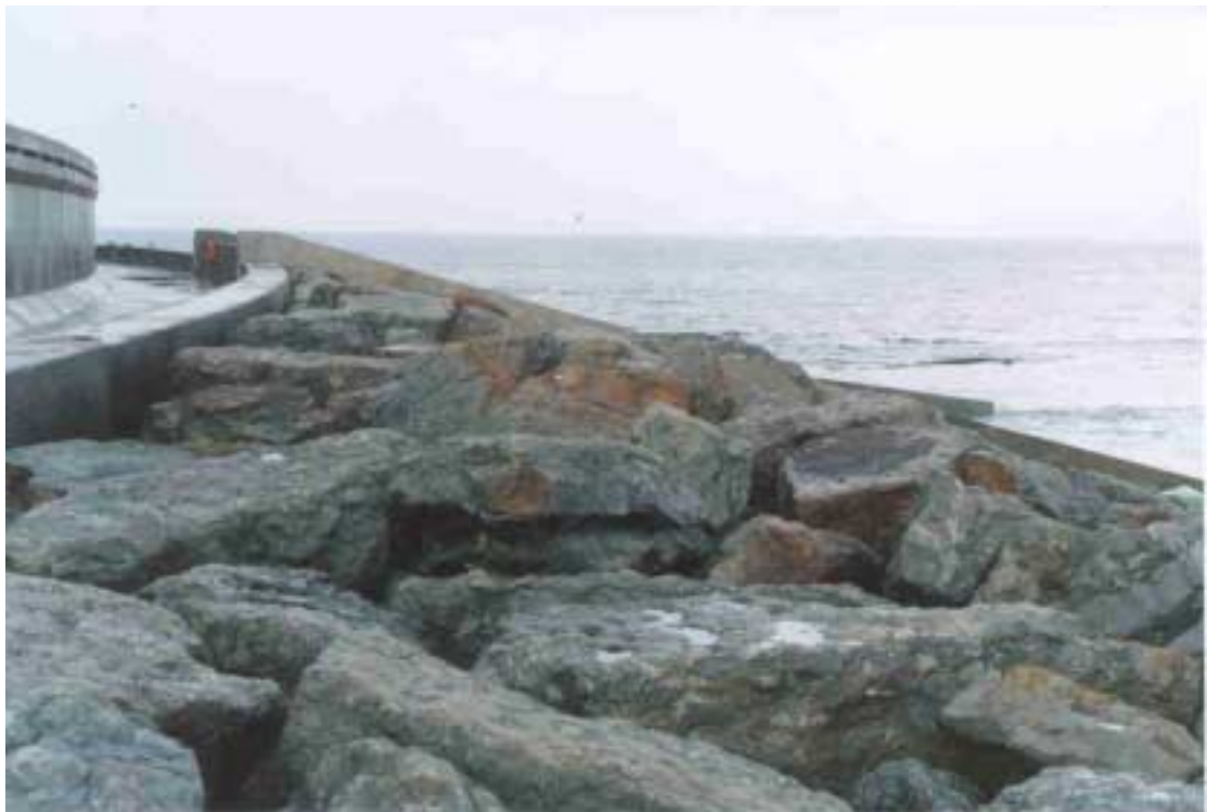
Plate 9.42 Defence No 58 Torness Power Station (Concrete Embankment protected by rock revetment)
