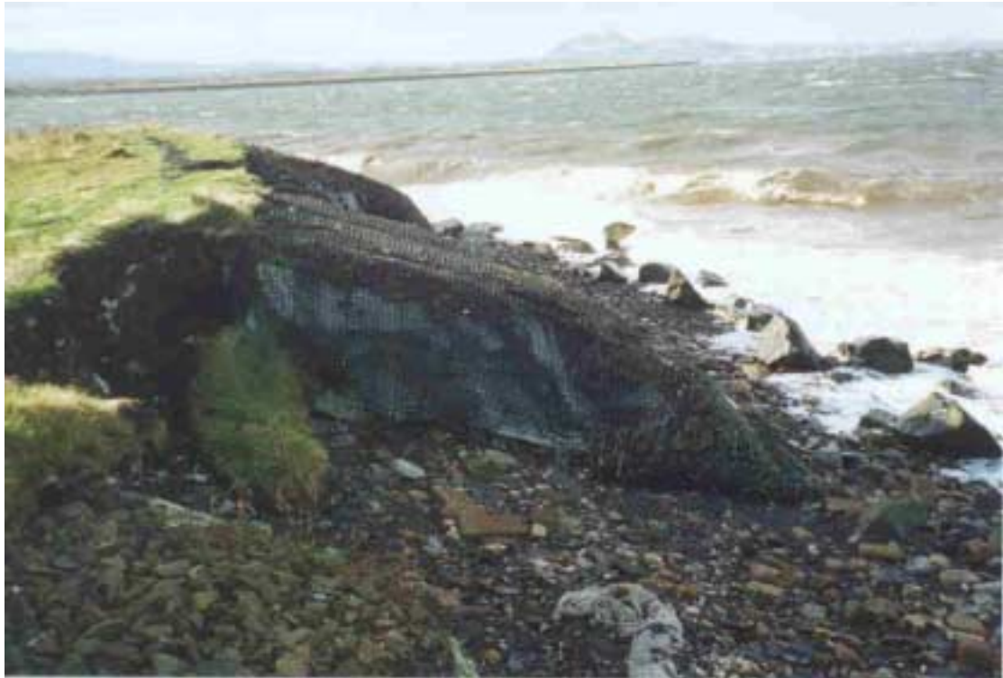
Plate 9.7 Defence No 10 Eroded Gabions at the Cast (Poor Condition)
