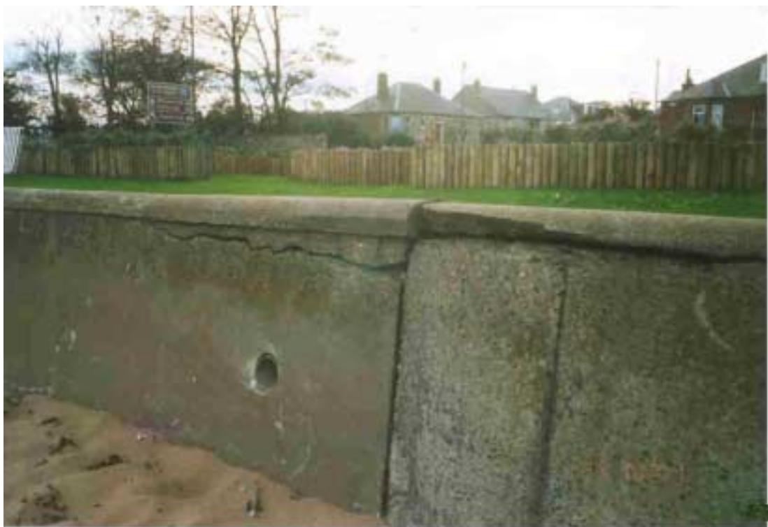
Plate 9.2 Defence No. 2 Concrete Seawall at Fisherrow Sands
