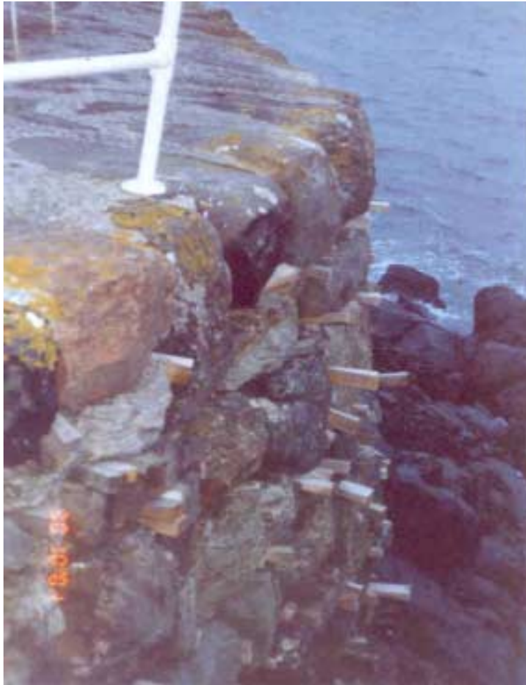
Plate 9.25 Defence No 33 North Berwick Harbour (Repairs to outer wall)
