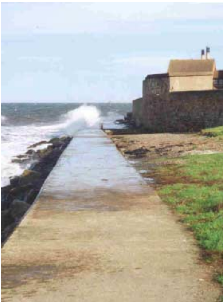
Plate 9.7 Defence No 10 Eroded Gabions at the Cast (Poor Condition)
