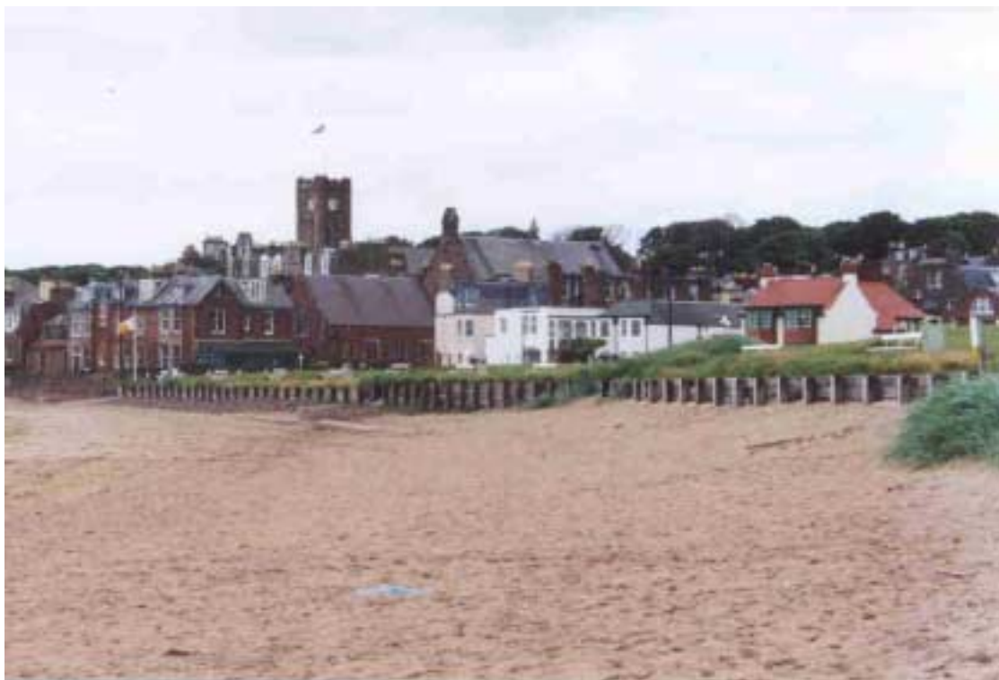
Plate 9.22 Defence No 30 North Berwick Bay, Timber Wall
