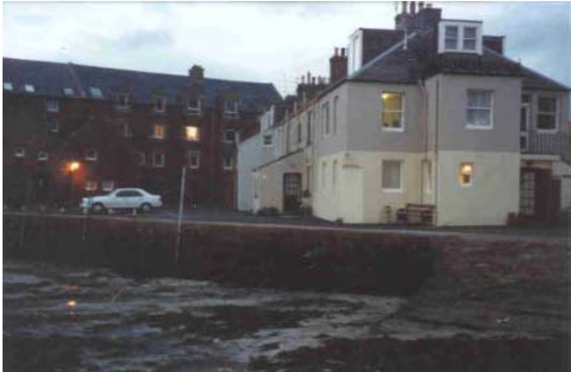
Plate 9.23 Defence No 32 North Berwick Bay, Low masonry wall
