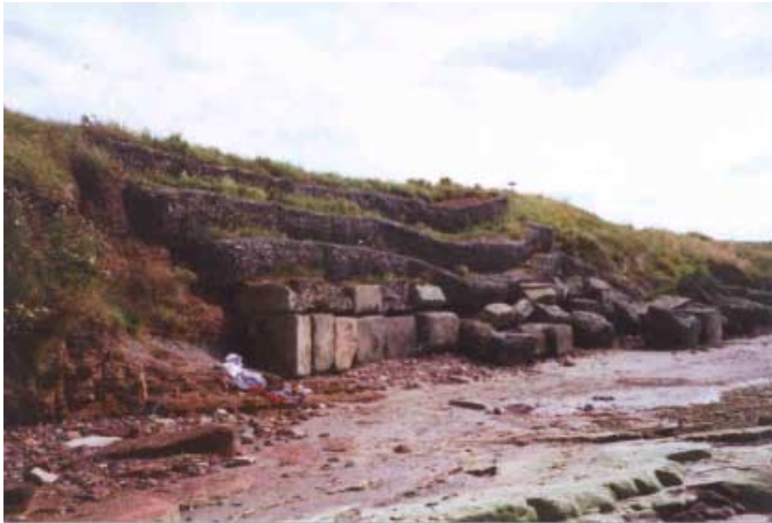
Plate 9.27 Defence No 39 Winterfield Golf Course, Gabions
