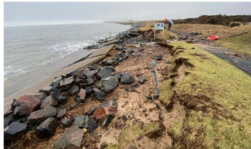
11. Re-exposure of vertical sleepers (former defences). Erosion above rock armour and loss of path, adjacent to the norther end of golf course. (282701,899474)
