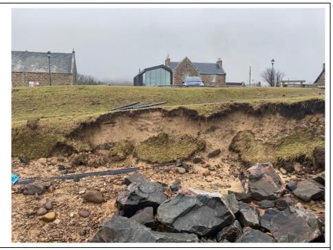
10. Erosion of land above damaged defences and damage to handrail. Debris extending inland. Note main sewer runs coast parallel here.
