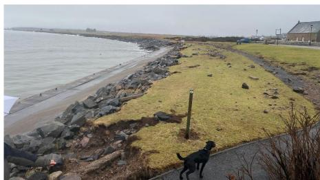
8. The orientation of erosion and the position of debris (thrown to west) confirm easterly waves. Church St. (282778, 899545)
