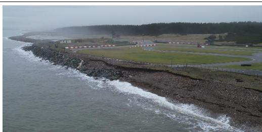
20. Southern extent of Kart Track defences washed out, exposing car tyres, which have been carried south into Loch Fleet NNR. Note erosional bight at southern end of Kart track caused by presence of defences (282111, 897668)
