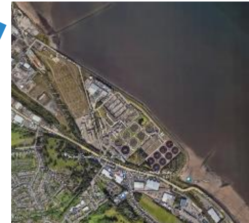
The Seafeld Wastewater Treatment Works (Responsible body: Veolia / Scottish Water)
