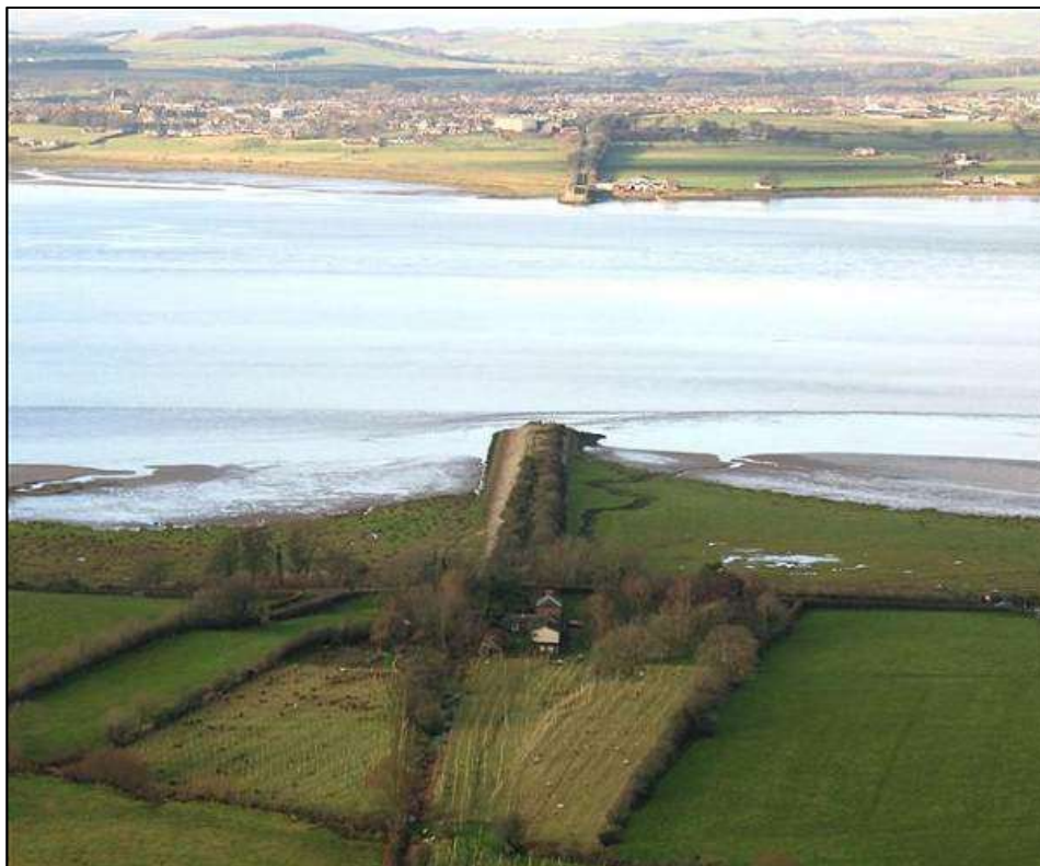
Figure 7.21: The Solway Junction Railway viaduct at Bowness on Solway, looking north toward its landfall at Annan ( http://www.visitcumbria.com/car/solway-junction-railway/ )
