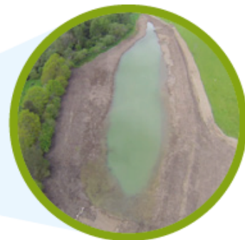
Flood retention pond at Kidston Mill
